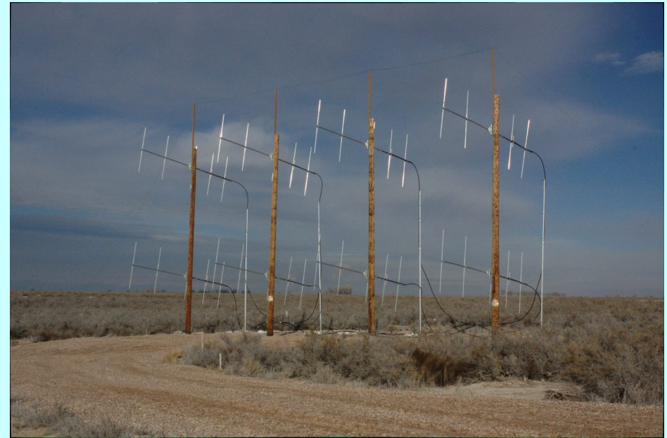
The TARA transmitter array.
