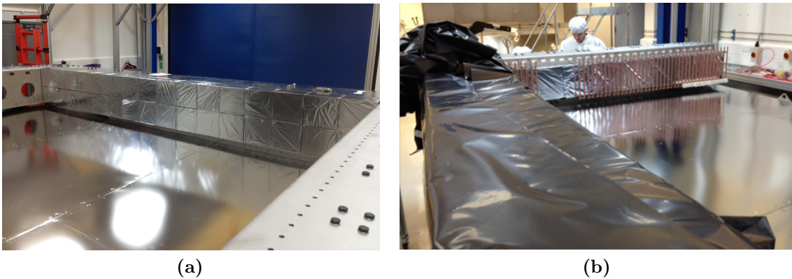
Figure 9.3.: Photos of SuperNEMO construction, showing the installation of optical modules into the first C-section. (a) shows two rows of 16 wrapped scintillator blocks attached to the frame and (b) shows the tracker cell support structure in front of another row of larger optical modules.
