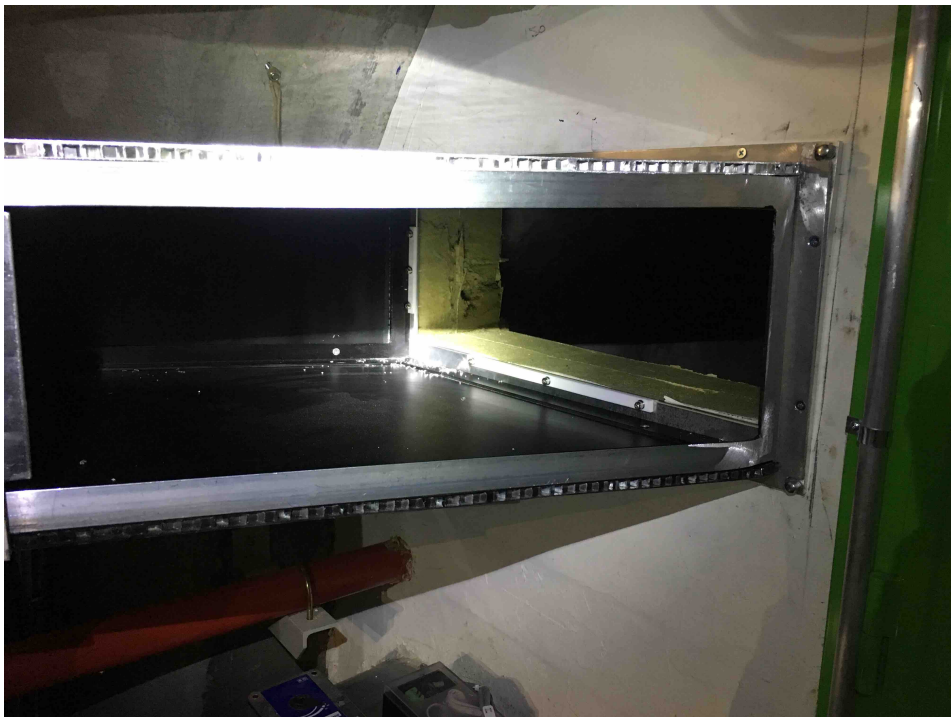
(d) Fire window and protective housing with the side panel removed.
